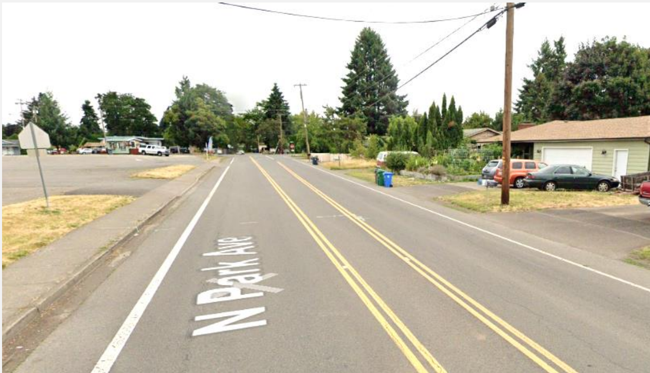
Figure 4. North Park Avenue Conditions
